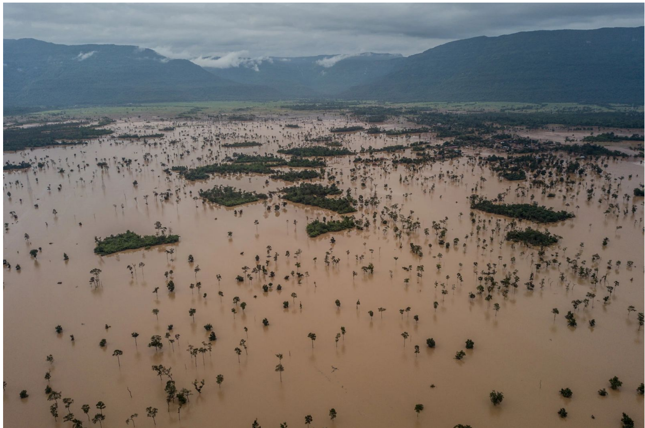
Fig 7- Floods due to the dam break (Source: https://www.nytimes.com/2018/07/26/world/asia/laos-dam-collapse.html )
