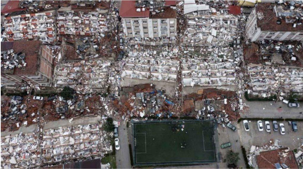
Figure 15: Pancake collapsed buildings in Hatay (Credit: IMO 26 )
