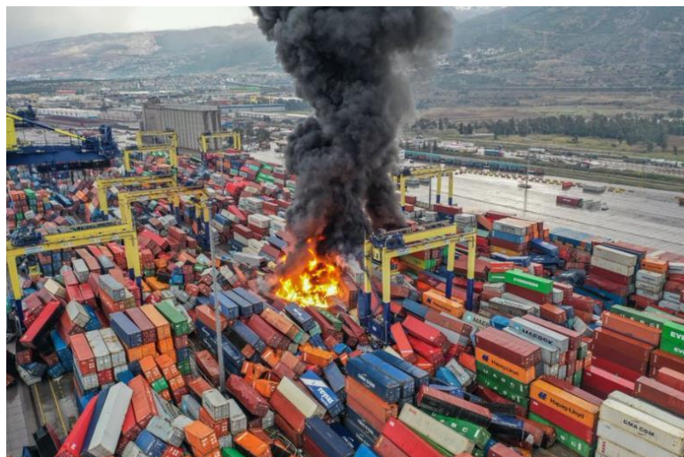
Figure 11. View of the container fires at Iskenderun port.
