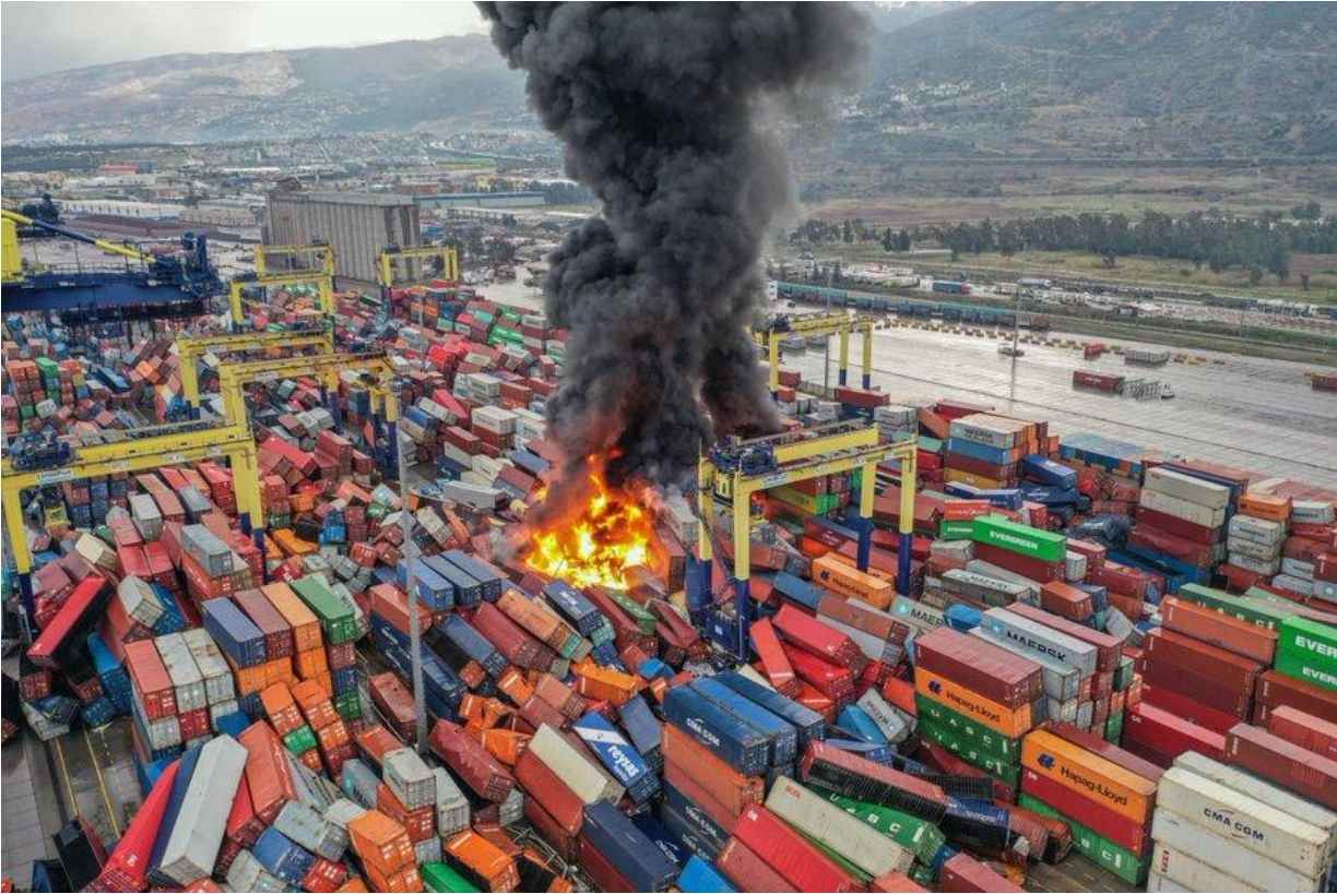
Figure 3 – View of the container fires at Iskenderun port.
