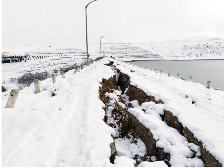
Figure 9: Longitudinal cracks on the Sultansuyu Dam. 7
