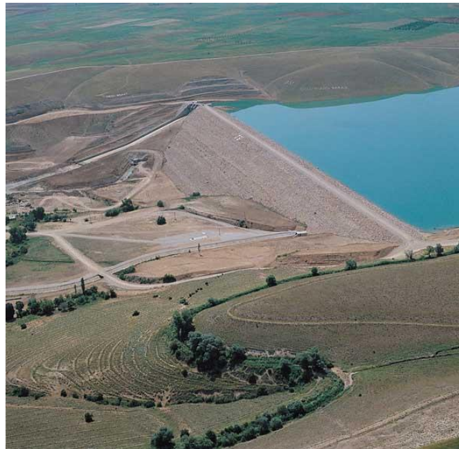
Figure 10: Image of the Sultansuyu Dam (source: Yüksel)
