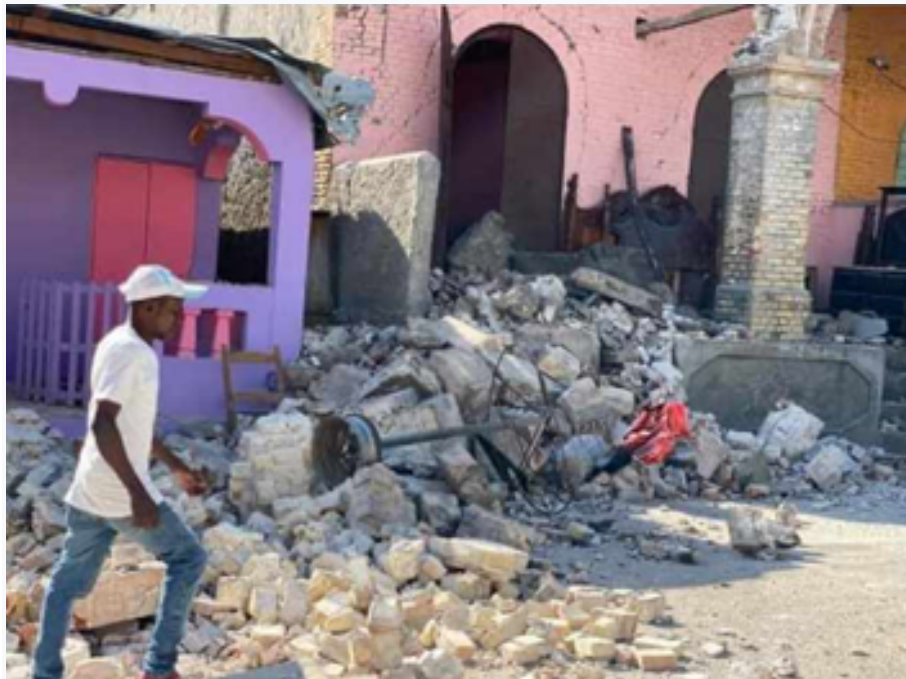
Fig. 12 - Damage due to the earthquake (source: private communication).
